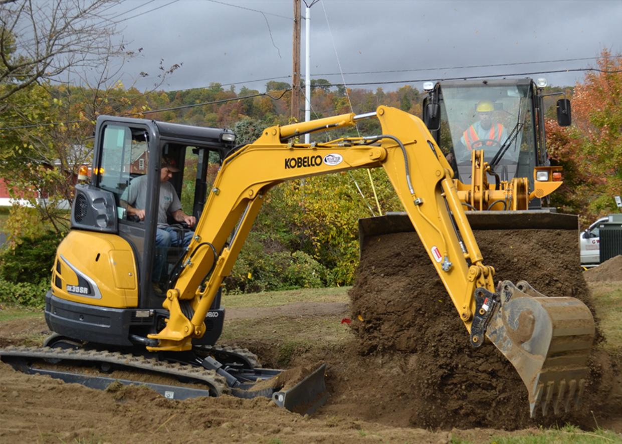
Photo Caption: GWS Contractors of South Brunswick, NJ, utilize the KOBELCO SK35SR for the removal and remediation of an old oil tank.
