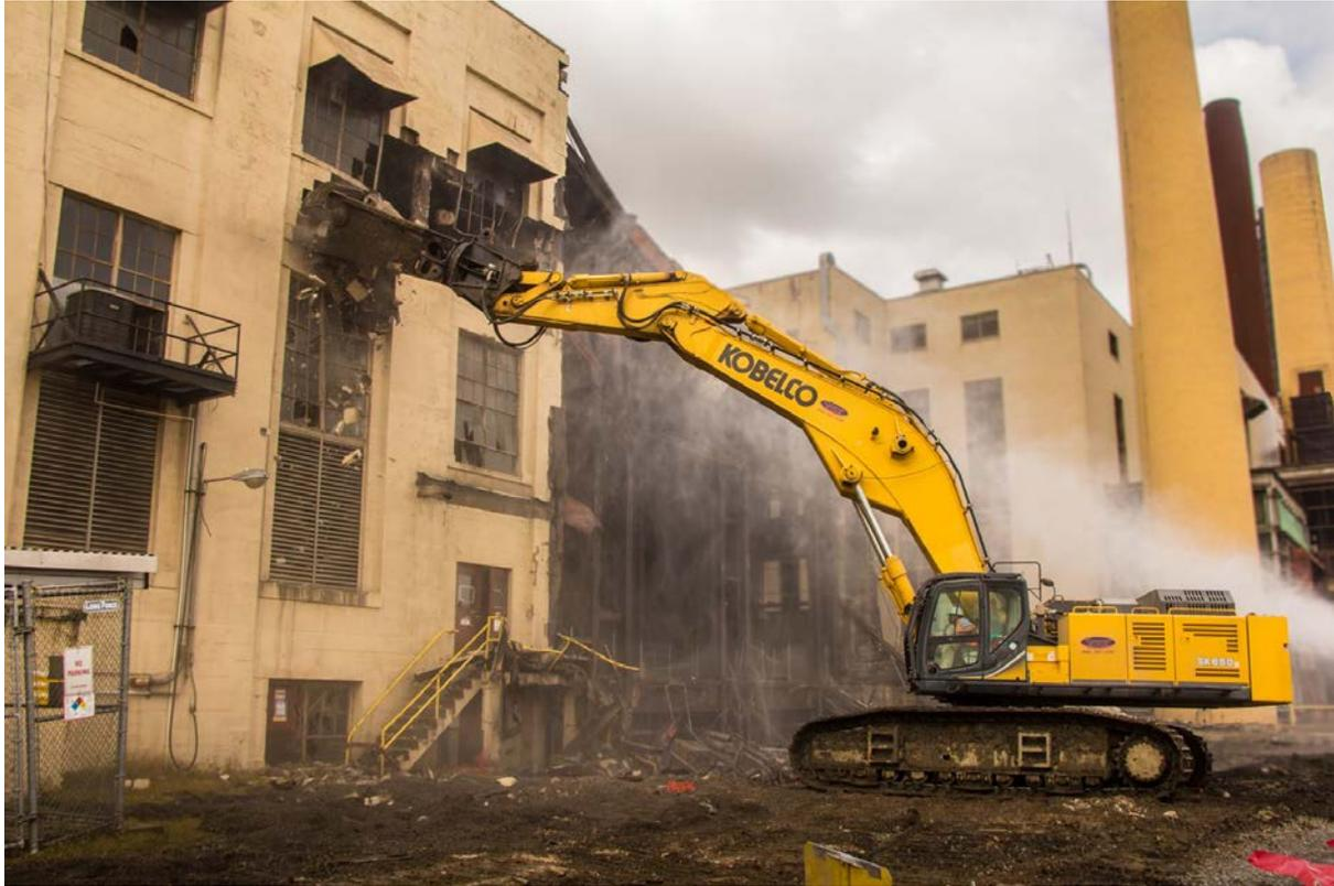
Photo Caption 1: KOBELCO's SK850 is being used by NorthStar to dismantle a majority of the Benning Road Power Plant in Washington, D.C.
