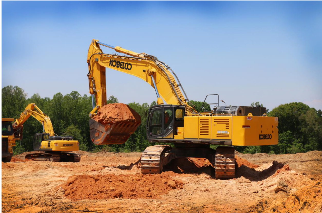
Photo Caption 3: KOBELCO excavators prepare the site for the company's new North American manufacturing facility.
