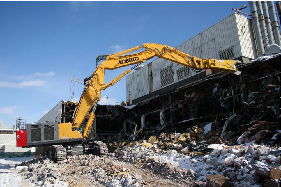
Photo Caption 2: The KOBELCO SK1000 working on site at the General Motors assembly plant in Oshawa, Ontario.
